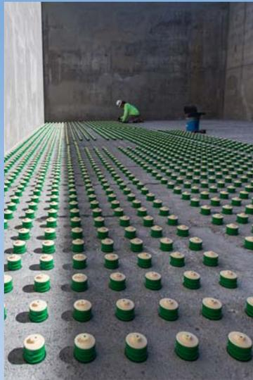
Monolithic Underdrain Filter Nozzles
