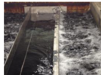
Ortho-Wash Media Retention Baffle
